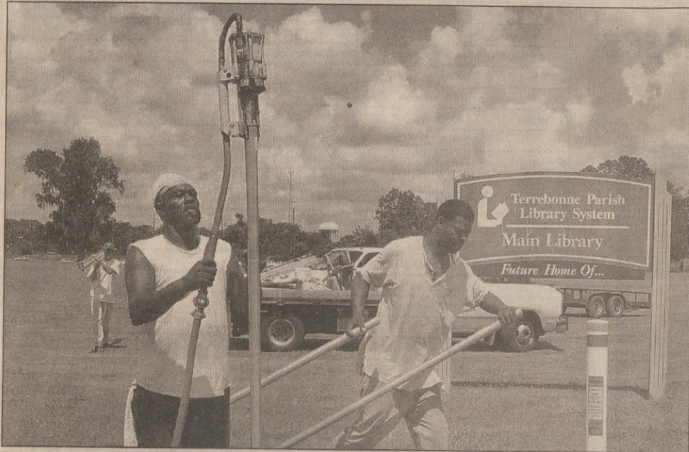
Bruce Harris, Sr., a construction worker for Tribble B Construction and Fence of Vacherie, uses an air compressed post driver to anchor a galvanized steel fence post into the ground, as his son Bruce Harris, Jr. helps out. Tuesday, September 4, 2001, marked the first day of construction of the new Terrebonne Parish Main Library.
